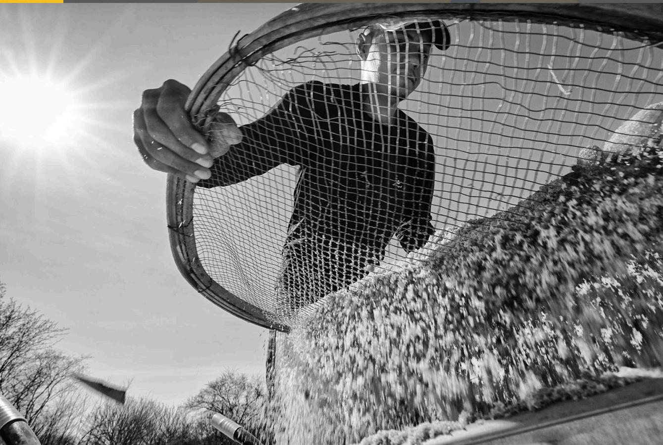
Construction of Cisterns Photography: Tadeu Vilani.
